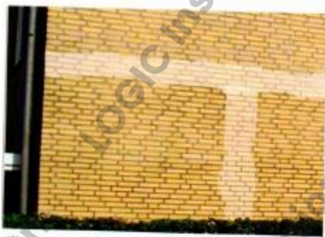
White smooth traces on top of overlapping silicon treatment on exterior after silicone treatment.
