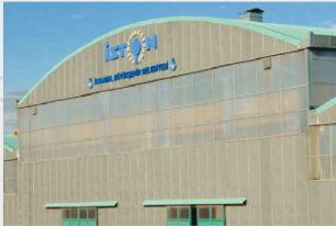
İSTON A.Ş Concrete Plant
